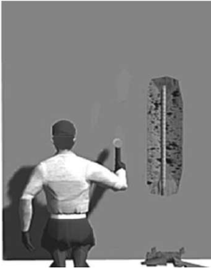
Removal of loose concrete
